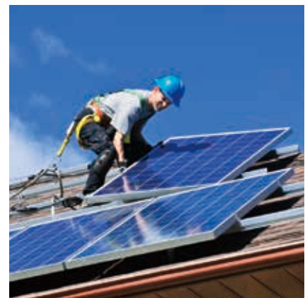
Perform load rejection testing of solar power systems
